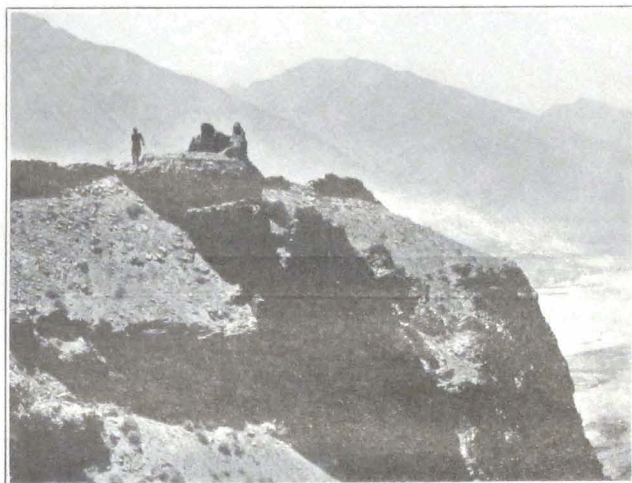
408. OUTWORK ON WEST FACE OF CIRCUMVALLATION, ZAMR-I-ĀTISH-PARAST.
