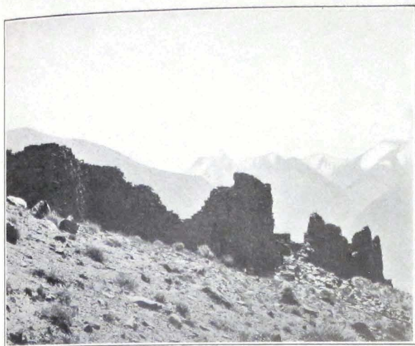
395. RUINED WALLS OF ZANGIBĀR FORT, WAKHĀN.
